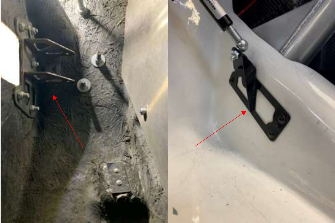
Figure 10: Door hinge bracket and hand door damper support bracket
